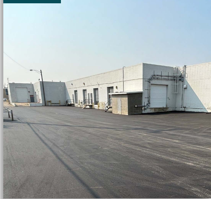
PAVED YARD AREA
