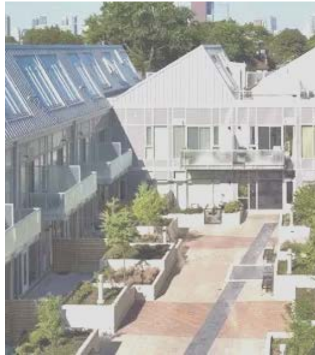
PRINTING FACTORY LOFTS
