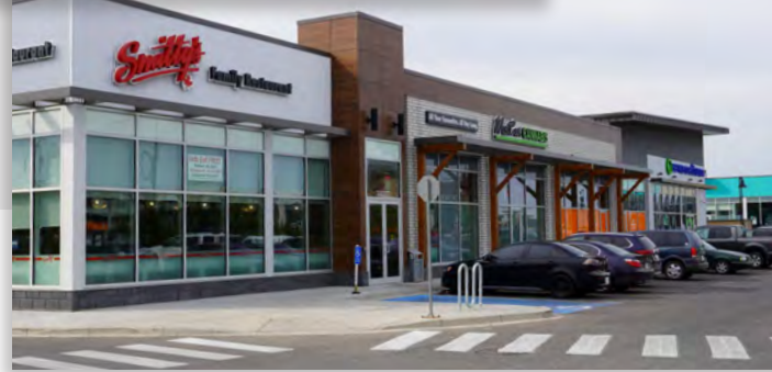
Fully fixtured quick service restaurant
